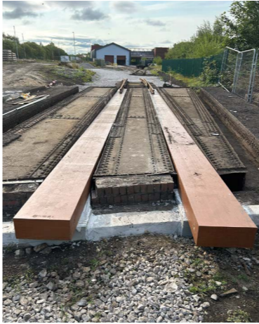
Above: The waybeams being positioned on the Otley Terrace bridge allowed the team to start the final push to connect the track to DLW.
