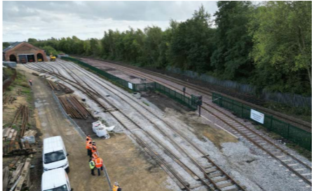
Above and right: The finished result, impeccably laid and finished track connected to the Network Rail siding, which allowed Tornado to be the first steam locomotive to enter the DLW yard from the main line.
