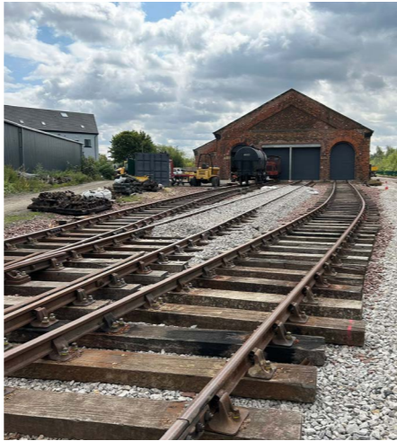
Track is extended to the Whessoe Road engine shed.
